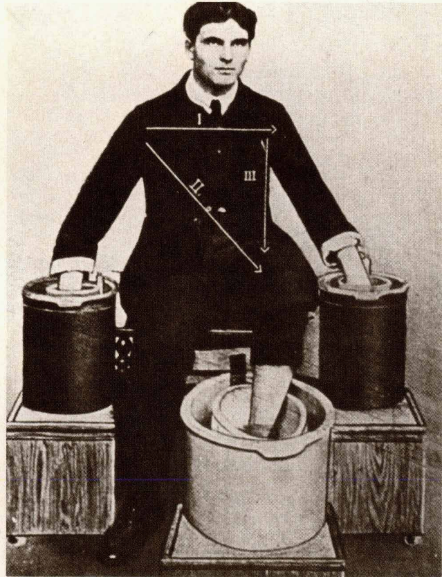
Fig. 1. Early ECG measurements required putting the subject's limbs into buckets of saline solution to make sufficient electrical contact for detecting the electrical activity of the heart muscles on a string galvanometer (source of picture unknown). The Roman numerals indicate three of the commonly recorded levels. They are derived by taking voltage differentials referenced to the right leg. That is: I = left arm - right arm, II = left leg - right arm, and III = left leg - left arm.
